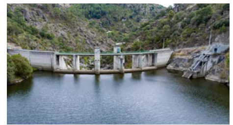
Hydropower Sagres, Portugal 21 plants, commissioned 1951-2006
